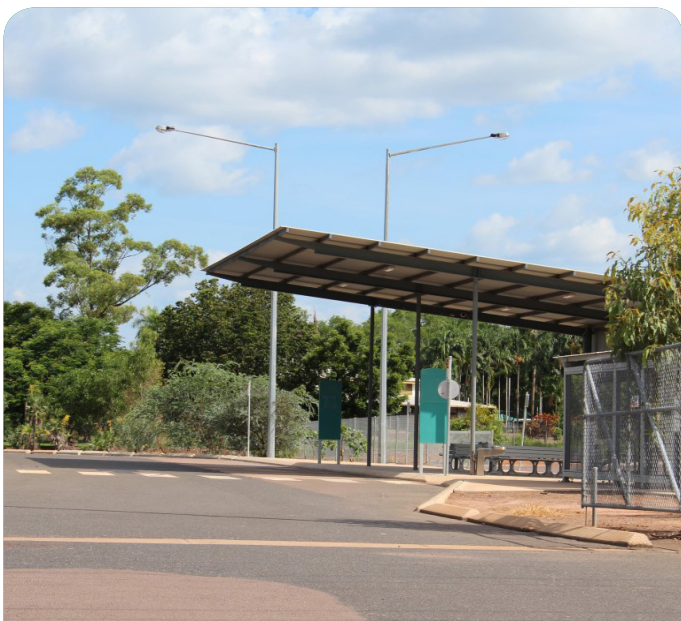
Humpty Doo Bus Interchange
