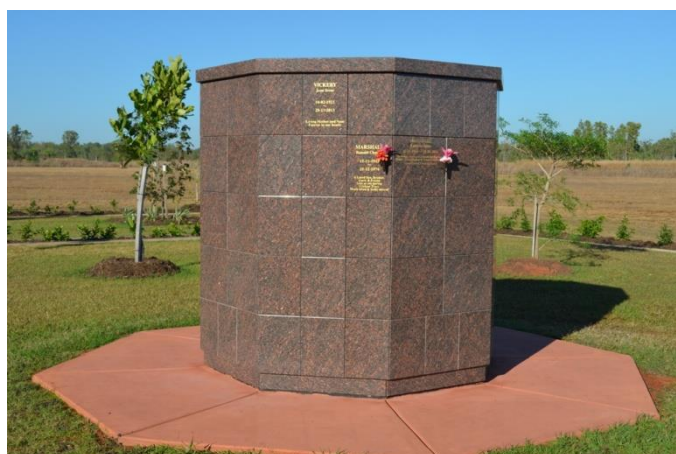
The Columbarium is a newly built cylindrical granite structure where the urn is placed inside the niche face and the niche face is etched with your memorial words.
