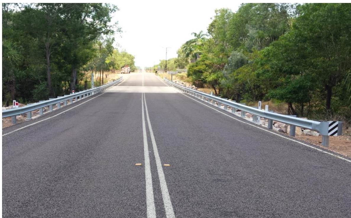
Leonino Road Culvert, Darwin River
