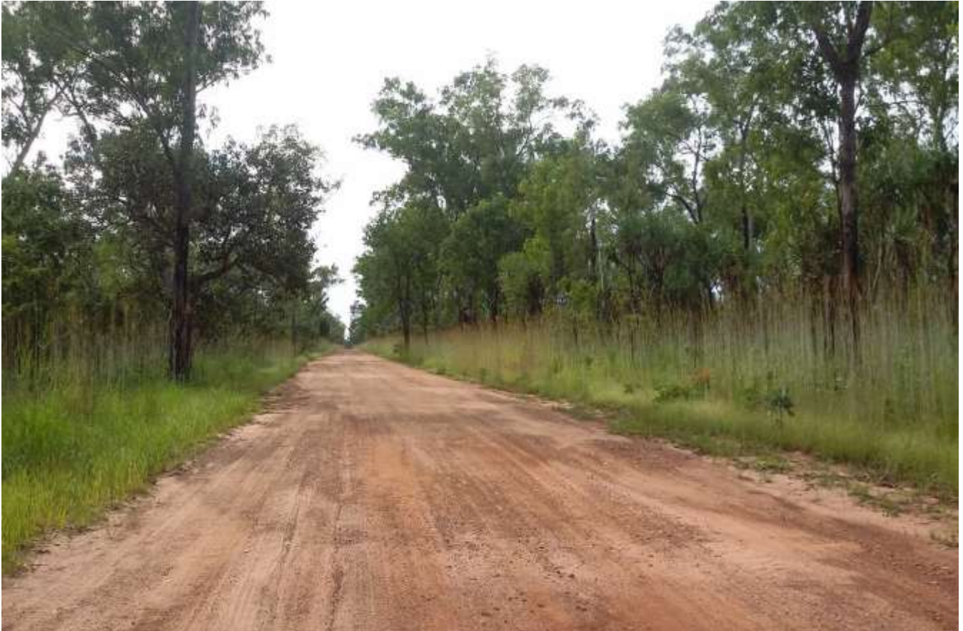
Figure 2 - Typical unsealed (gravel) road
